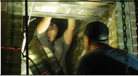
Inside the chimney on a makeshift platform, installing the bracket to hold the liner.
