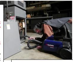
We vacuum out the flakes to keep the hot water heater going temporarily. It could quit for good at any moment.
