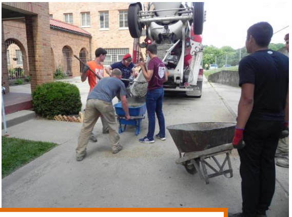
...Using wheelbarrows to move 3.5 yards of concrete.
