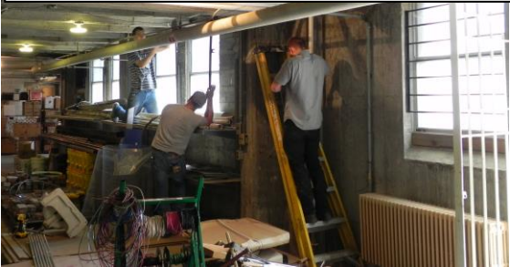
Volunteers from St. Mary’s completed many jobs, including moving outlets.
