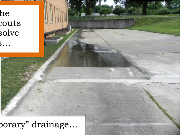
...Re-routing a blocked storm drain...
