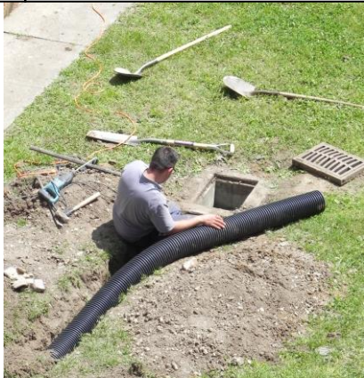
...Re-routing a blocked storm drain...
